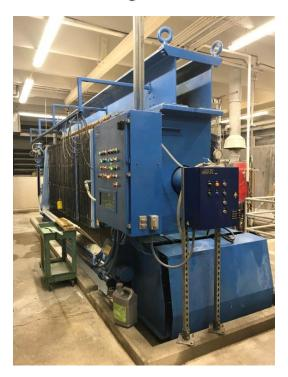
**Purpose:** To remove water from the lime sludge used to soften the drinking water. The WTP operates two of these filter presses which were installed in 1993.
