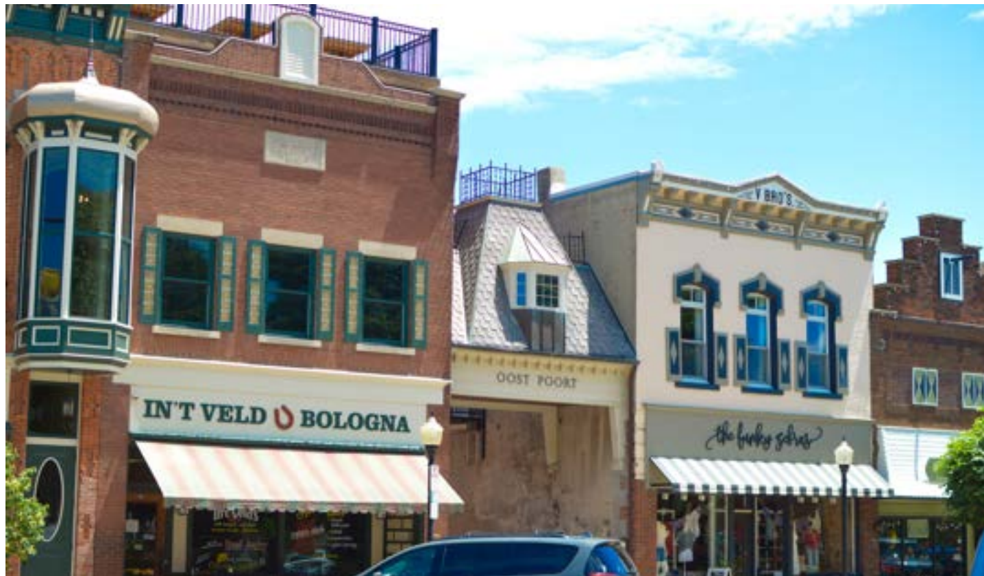
The design districts outlined correspond with the regions indicated on the district map on pages 20 - 21.
