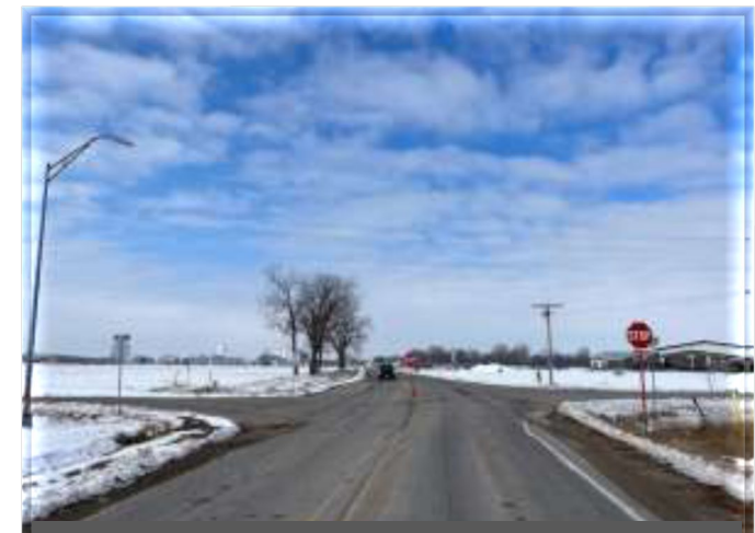
Oskaloosa Street - $1.85 M
