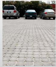
Rainfall soaks through permeable pavement and into the ground below in this parking area in west Des Moines, lowa.
