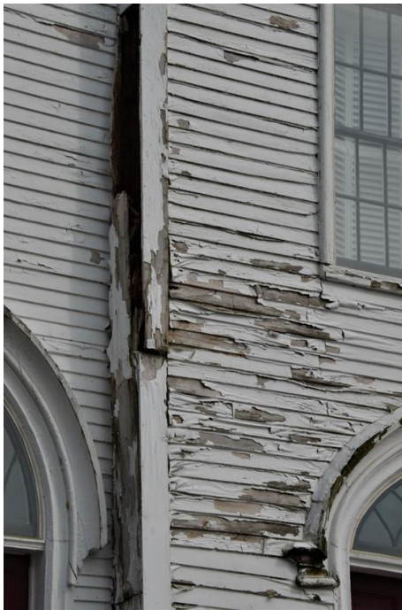
Depth of decay at northwest corner post, ground floor
