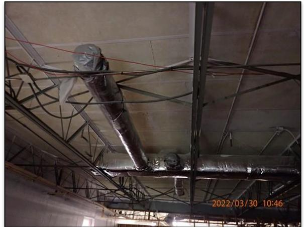
Figure (10) – HVAC duct above Room 4 covered with polyethylene sheeting.
