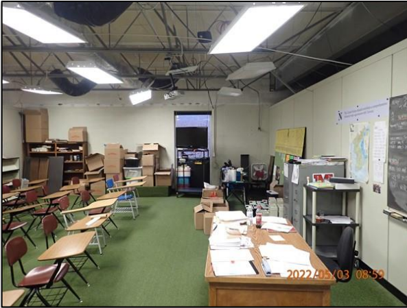
Figure (7) –Overview of Room 26.
