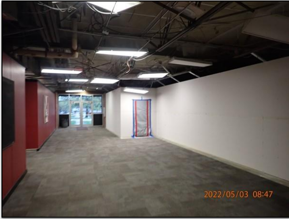
Figure (1) –Hallway outside Room 4 and Room 3.
