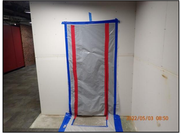
Figure (2) – Polysheeting covering door to Room 4.
