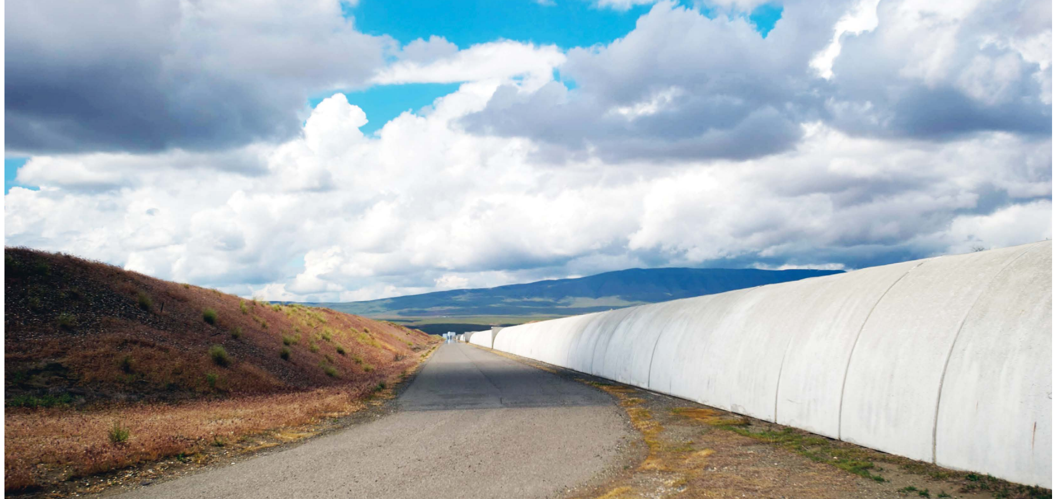
One of LIGO's Washington State Hanford's 'arms'. The "mid-station" (half-way to the end of the arm) is barely visible 2 km away. Photo by Kim Fetrow.
