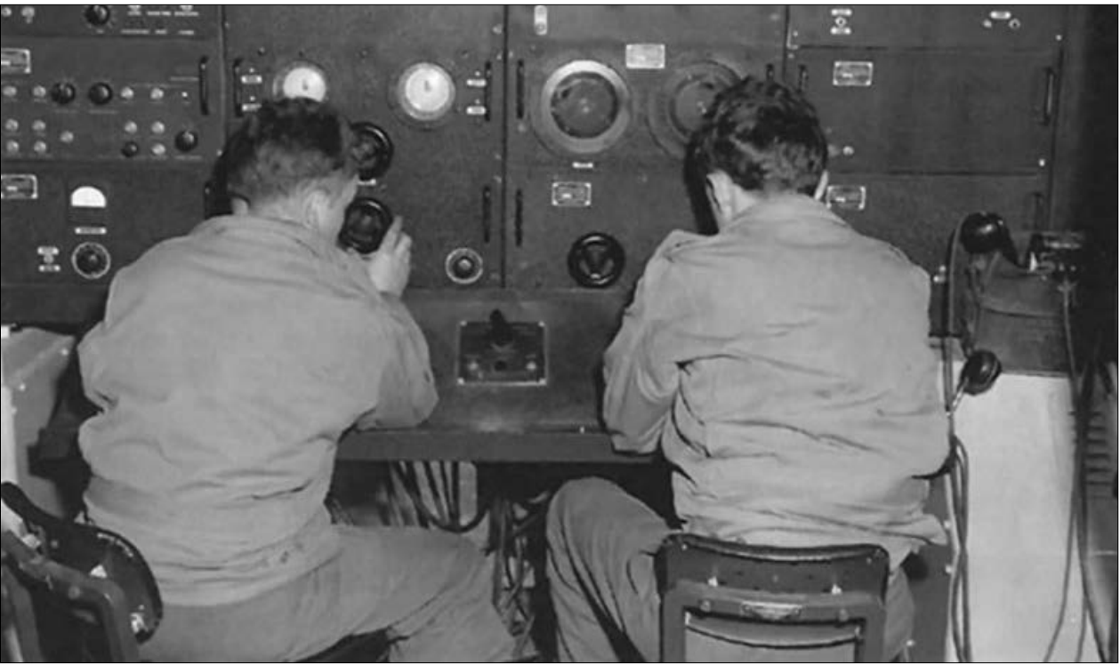
Interior view of the SCR 584 radar tracker that guided pilots to their targets. Contributed photo.
