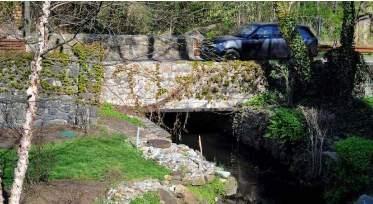
North Street Bridge - to undergo reconstruction. Contributed photo.
