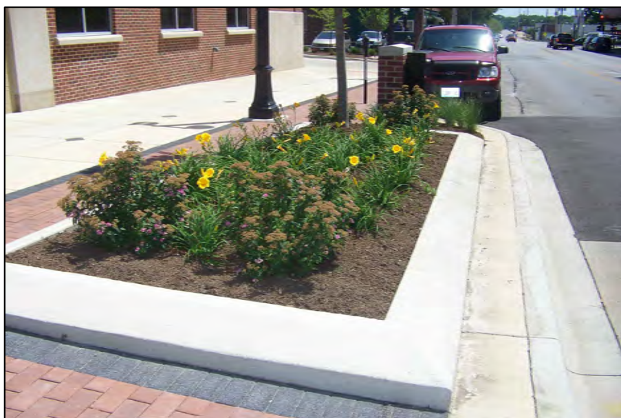
Plant Bed with Perimeter Curb to Protect Plants and Provide Adequate Soil Depth
