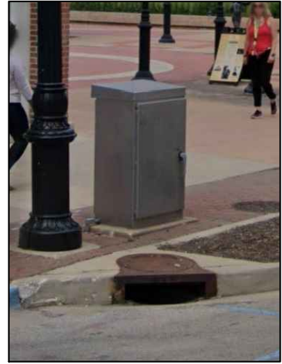
Wrap utility cabinets
