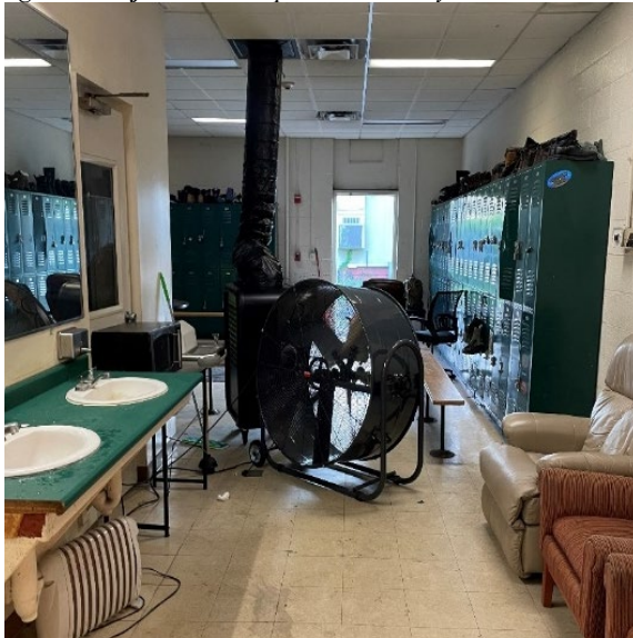
Figure 9: Before DPW improvements July 2024
