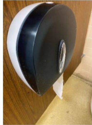
Figure 8: After DPW Repairs August 2024
