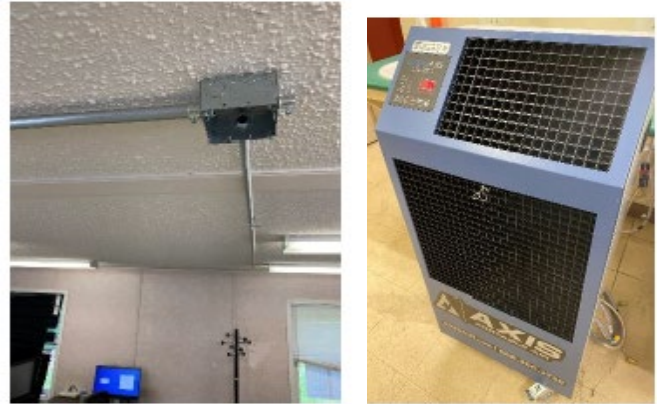
Figure 14: After DPW Repairs August 2024
