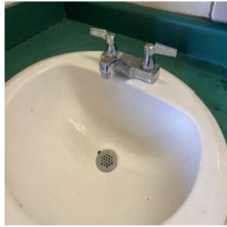
Figure 12: After DPW Repairs August 2024
