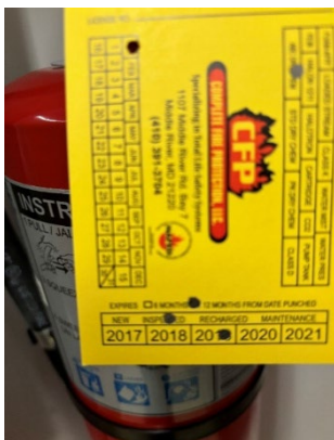
Figures 4 & 5: Expired (2019) fire extinguisher and fire alarm system control pad from 2024 BCFD inspection
