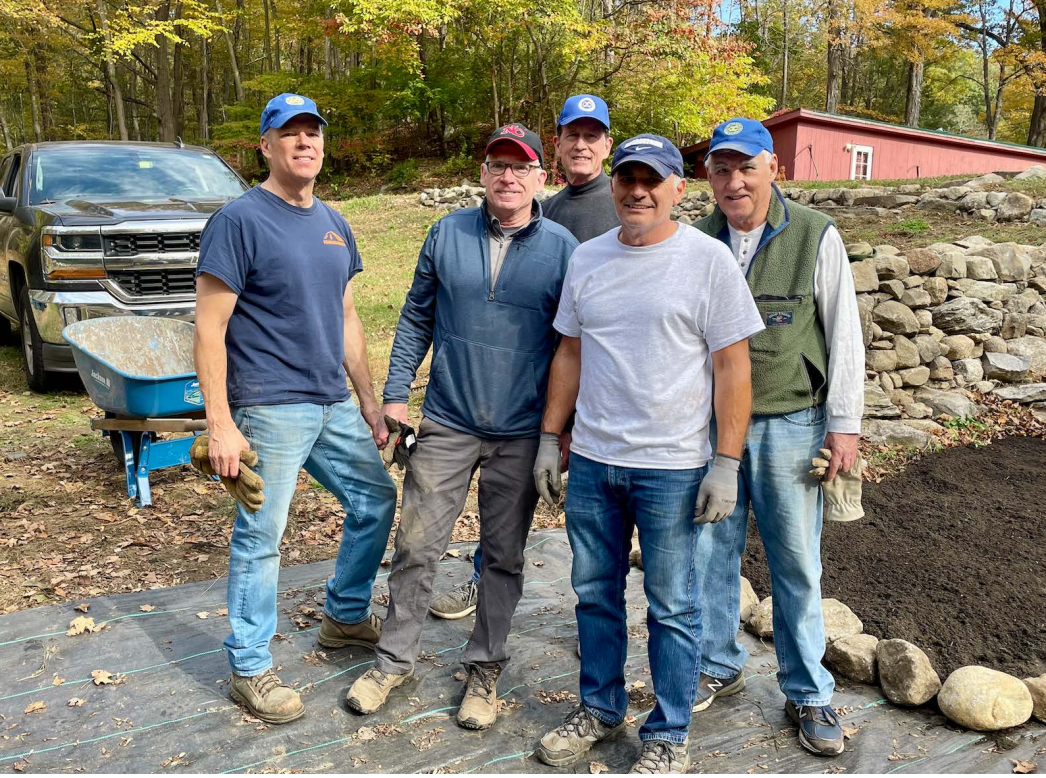
Several Exchange Club volunteers take a break from their labors at the New Canaan Land Trust's Grupes House during their Day of Service, showing the new pollinator garden they helped build, with its fieldstone border, behind them. Photo Credit: NCLT
