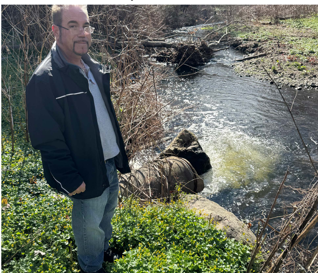
Waste Water Plant Superintendent Nick Colabella at the end of the line: The pipe from which cleansed water is discharged into the Fivemile River.
