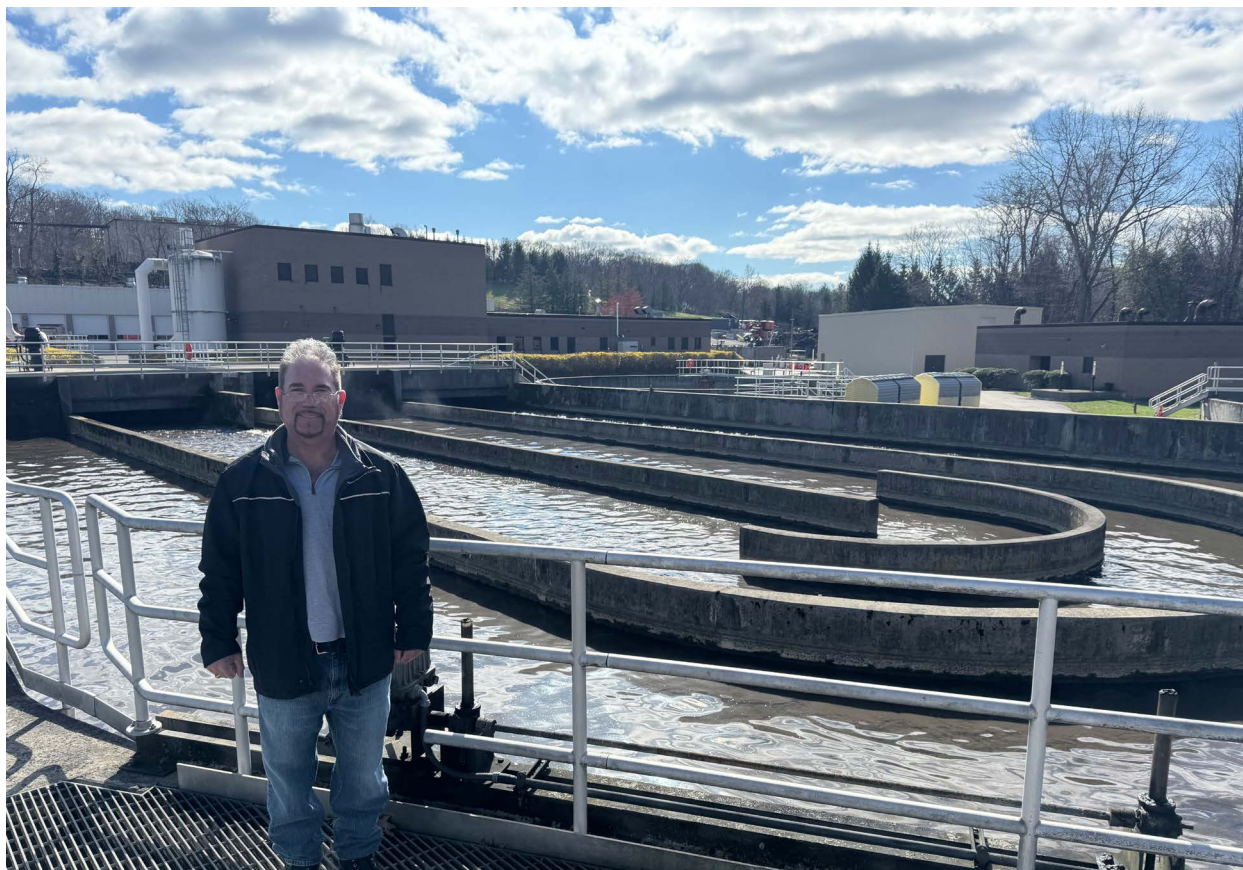
Waste Water Plant Superintendent Nick Colabella at the carousel tanks, one of the steps where waste water is processed and cleaned.
