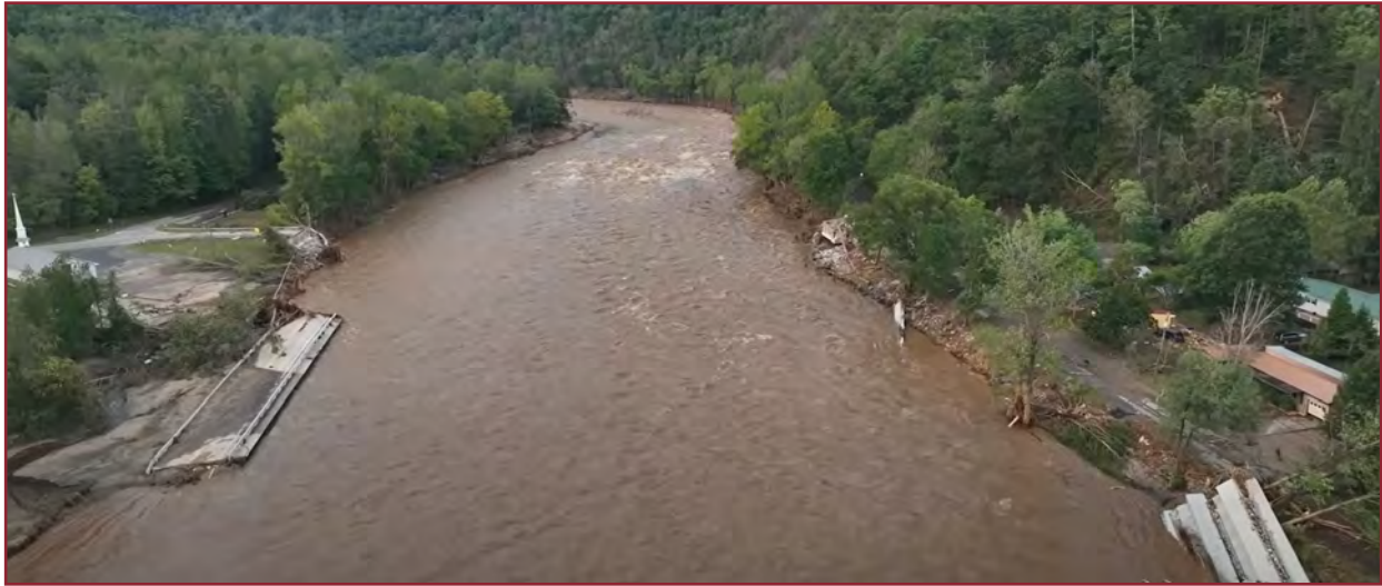
Remnants of Chestoa Bridge following Tropical Storm Helene
