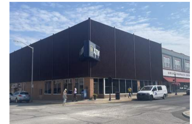
Pockets of non-historic facades and varied materials
