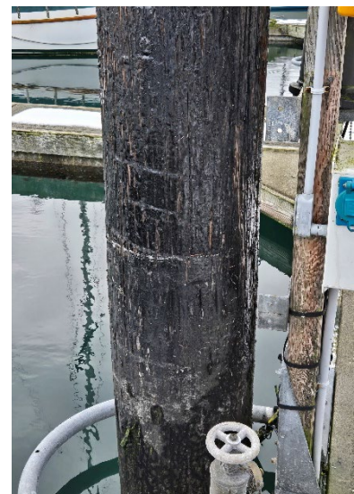
Figure 66. Piling at John Wayne Marina showing wear and tear from the metal piling loop during previous high tide events. (WA EMD)
