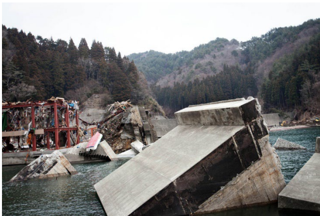
Figure 71: The Kamaishi breakwater, which failed during the 2011 Japanese tsunami (NY Times).
