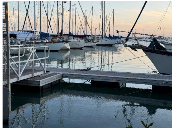
Figure 58: Docks built on floating blocks in Honolulu, Hawaii (WA EMD)
