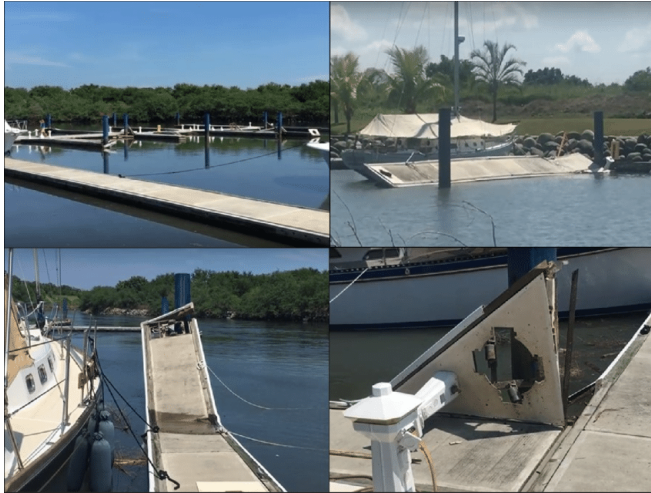
Figure 62: Dock damage in Marina Chiapas after the 2017 earthquake and tsunami. (Maria Teresa Ramirez-Herrera, 2017)
