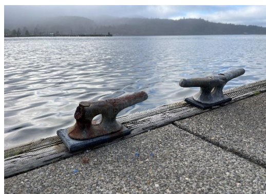
Figure 57: Broken cleat in Neah Bay along Dock A (WA EMD)
