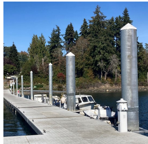
Figure 644. Piles in Eagle Harbor, City of Bainbridge Island, WA that incorporated SLR into their design. (WA EMD)
