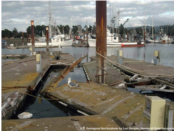
Figure 59: Broken docks in Crescent City, CA from the 2006 Kuril earthquake (USGS 2006).
