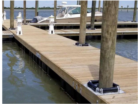
Figure 65: Floating docks with square pile guides for each piling (americanmuscleddocks.com).
