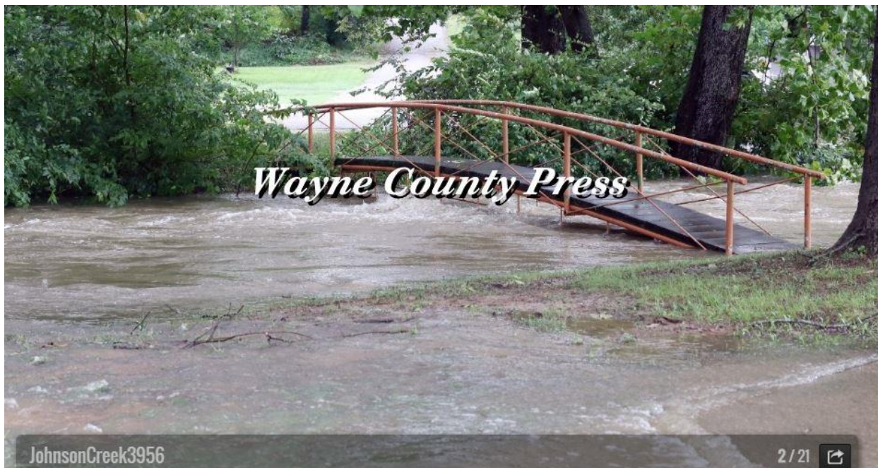
Johnson Creek just below the breached dam at Lakeside Park September 8, 2018
